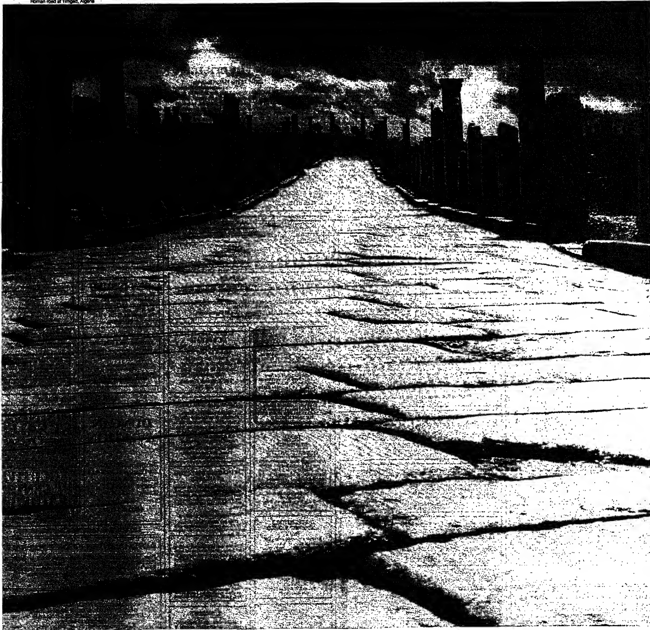
Roman road at Timgad, Algeria
